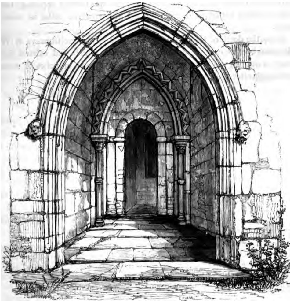
PORCH, WEST BARSHAM.
